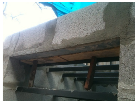
14. Timber formwork pieces supported under front besser bricks to hold concrete in place.
