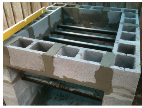
11. Could fill the besser bricks with concrete which prevents movement and reduces cracks in the mortar so I have been told. Also could put reinforcement bar inside the bricks. I didn't. Mine's still standing 😊
